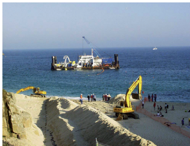
Figure 40. Submarine cable installation works in the coastal zone from BMH to low water mark. Source: www.ldravocean.fr.
