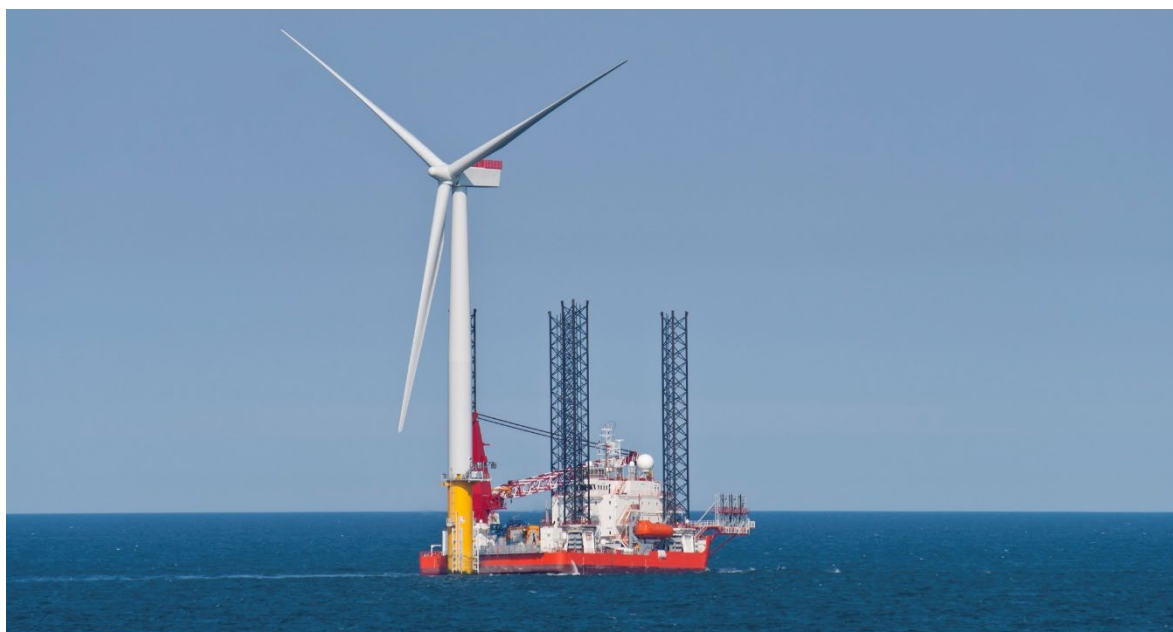
Figure 15. Offshore wind turbine being constructed, Norfolk, UK. Credit: iStock (user: DJMattaar).
