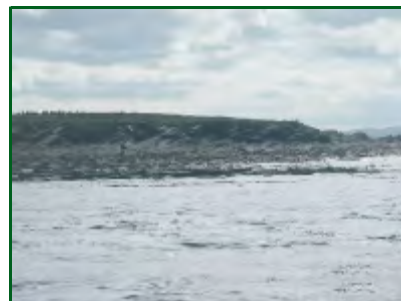
8 Broken bedrock cliff running to outcrop.
