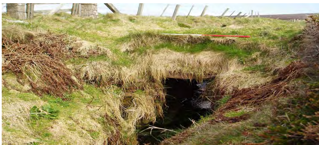
Plate 7.1 19th Century stone footbridge
