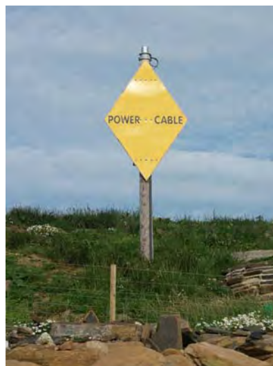
Plate 3.2 Cable marker board
