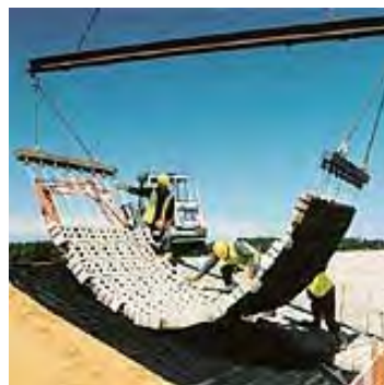
Plate 3.1 Armoflex concrete mattress
