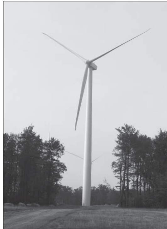
Figure 1. A wind turbine shown in a “feathered” position during a curtailment experiment designed to reduce bat fatalities at a wind facility in south-central Pennsylvania. (Photo courtesy of Edward Arnett)
