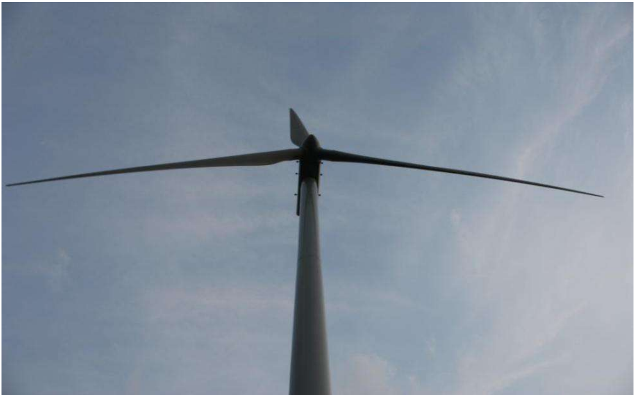
A wind turbine with six deterrent devices shown (3 mounted on each side of the nacelle; M. Baker, Bat Conservation International).
