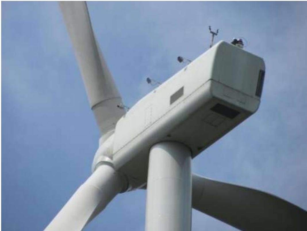
Deterrent devices attached to the nacelle of a wind turbine at the Locust Ridge Wind Farm in Pennsylvania (E.B. Arnett, Bat Conservation International)
