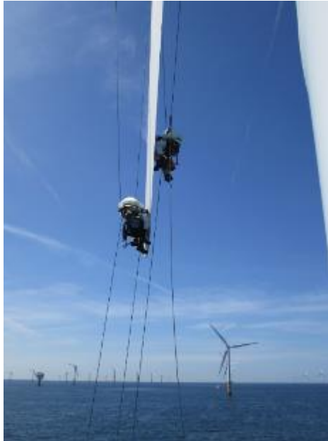
Figure 7: Rope workers at work on BW
