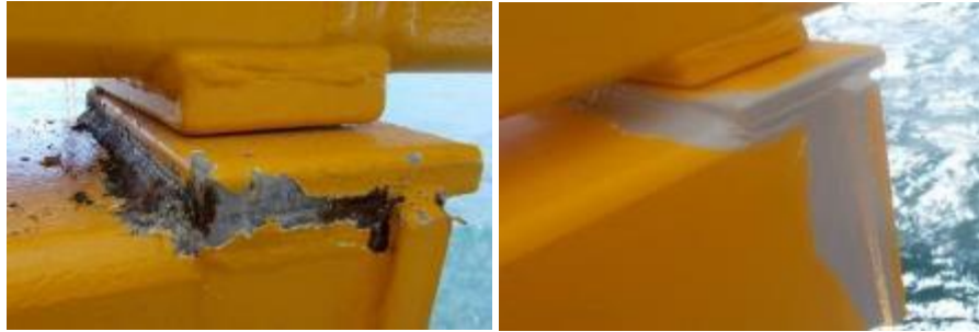
Figure 10: paint repairs foundation
