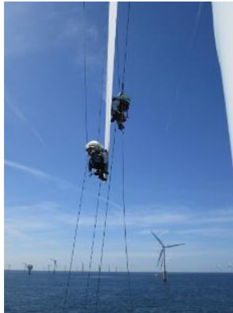
Figure 8: Rope workers at work on BW.
