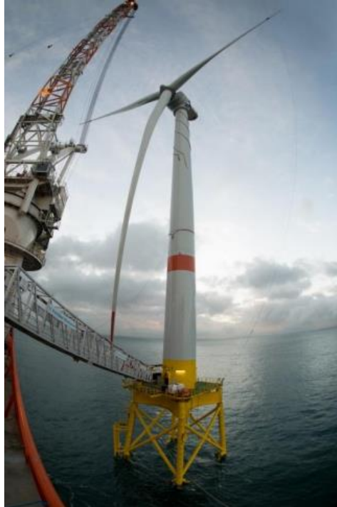
Photo 1: Alstom Haliade wind turbine
