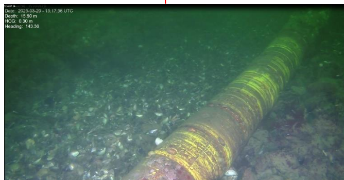
Figure 1: Monopile, cable protection system and scour protection in Anholt Offshore Windfarm (ROV pictures)
