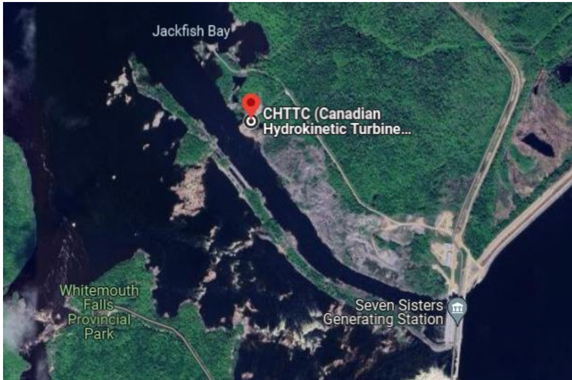
Figure 2: Aerial view of the Canadian Hydrokinetic Turbine Test Center (CHTTC) located near the Seven Sisters Generating Station. The CHTTC, marked by the red pin, is situated in a strategic position for testing hydrokinetic turbines, with proximity to both Jackfish Bay and Whitemouth Falls Provincial Park. The site offers a controlled environment with optimal flow conditions for turbine performance evaluation and research.
