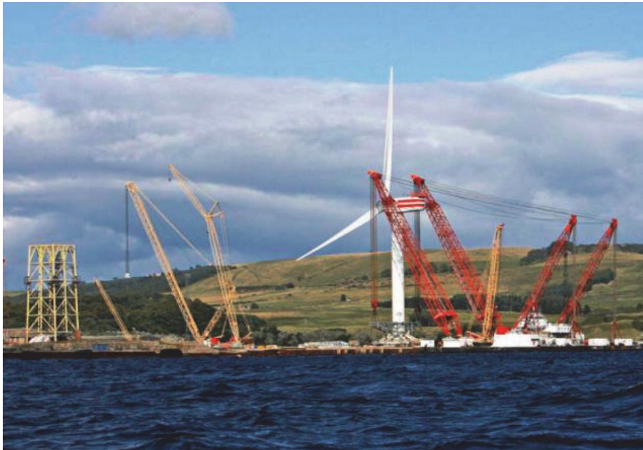
Figure 31: Wind turbine during construction Source: Simmonds & Dolman (2008) in Evans (2008)
