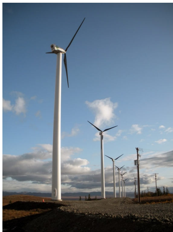
Figure 8. Unalakleet Valley Electric Cooperative installed six Northwind 100 turbines in November 2009. As of November 2016, the wind farm had generated 7 million kilowatt-hours of power and reduced fuel use in the remote Alaskan community by 70,000 gallons annually. Photo by STG Incorporated, NREL 16797
