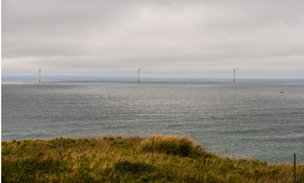
Figure 15. The Block Island Wind Farm (as seen from Block Island, Rhode Island) is the first U.S. offshore wind farm. Photo by Dennis Schroeder, NREL 40396
